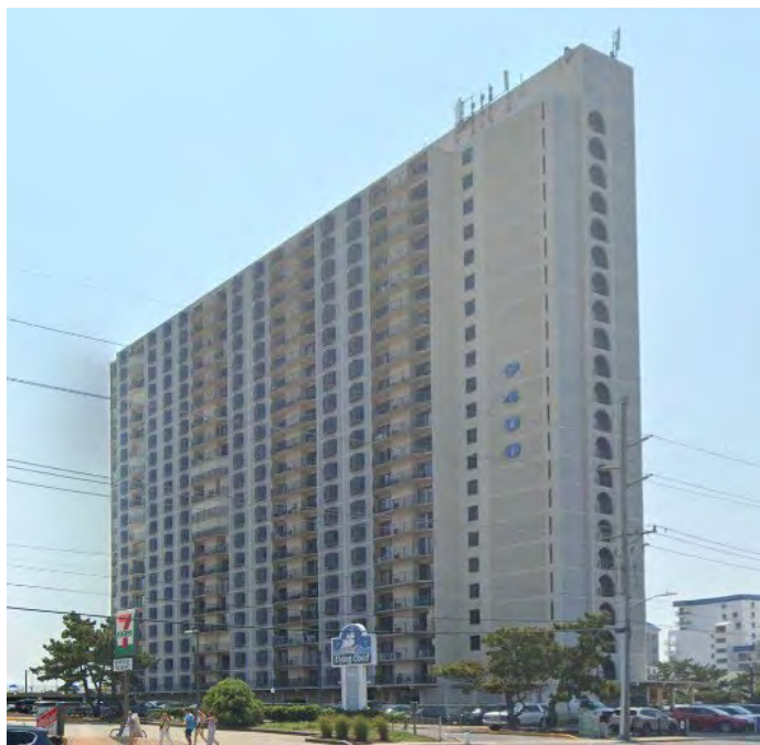
Photograph 3 – North elevation of the building.
