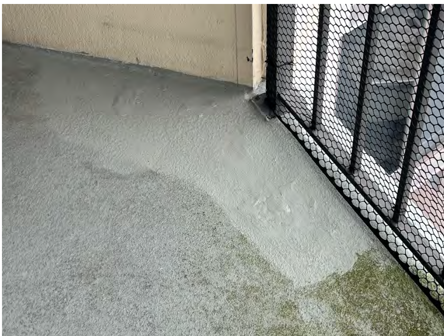
Photograph 8 – Balcony coating repair.
