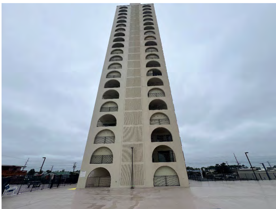
Photograph 4 – East elevation of the building.
